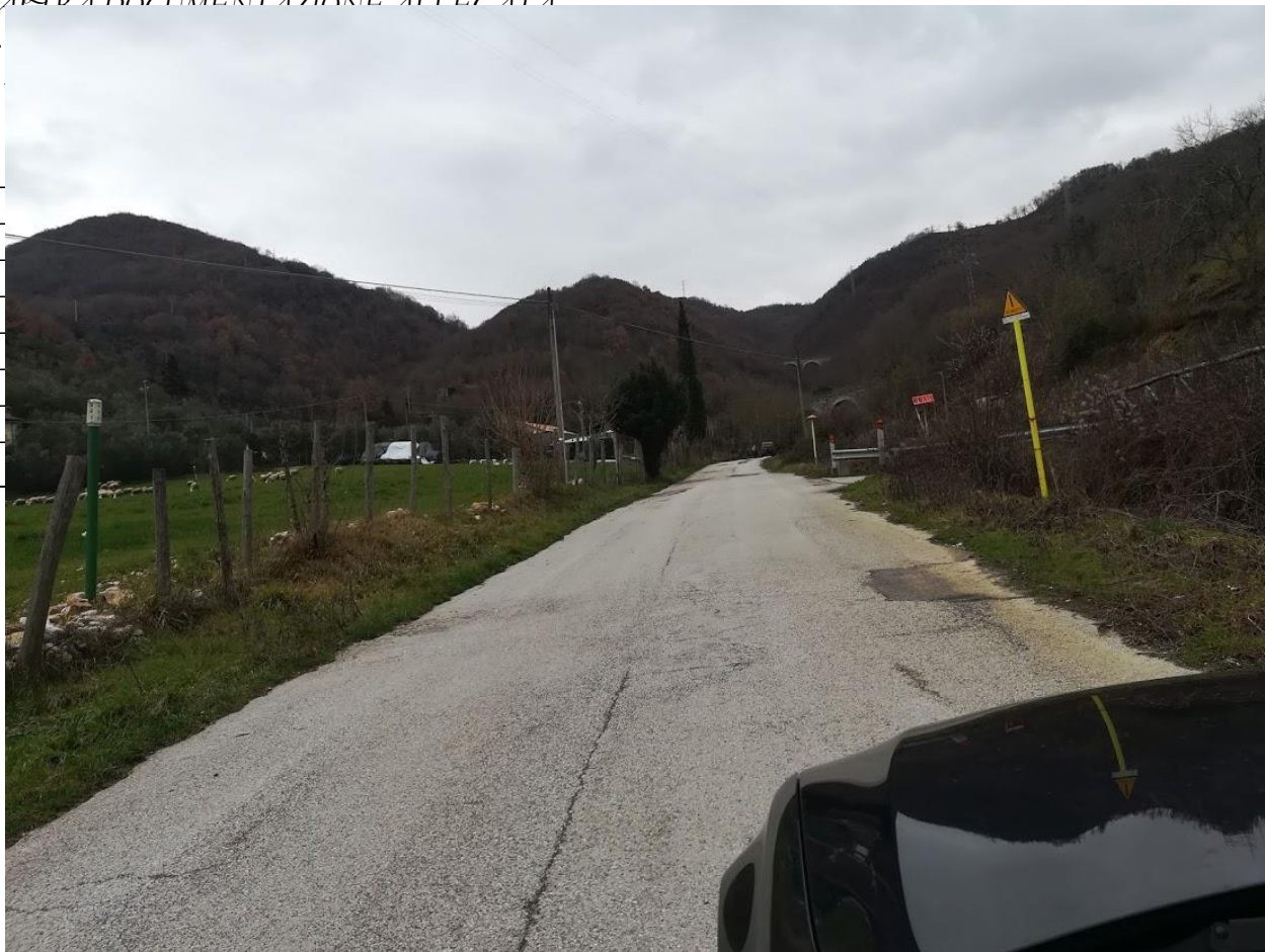
A first-person perspective from the driver's seat of a car, looking down a narrow, two-lane paved road. The road surface is light-colored and shows signs of wear and cracking. On either side of the road, there is a mix of green grass and bare, brownish trees and shrubs, suggesting a late autumn or winter setting. In the distance, a small village is visible, nestled in a valley. The village includes several houses with light-colored roofs and a prominent church with a tall, dark spire. The background is dominated by large, rounded hills or mountains covered in dense, dark vegetation. The sky is filled with heavy, grey clouds, creating an overcast atmosphere. The bottom of the frame shows the dark, curved hood of the car.
